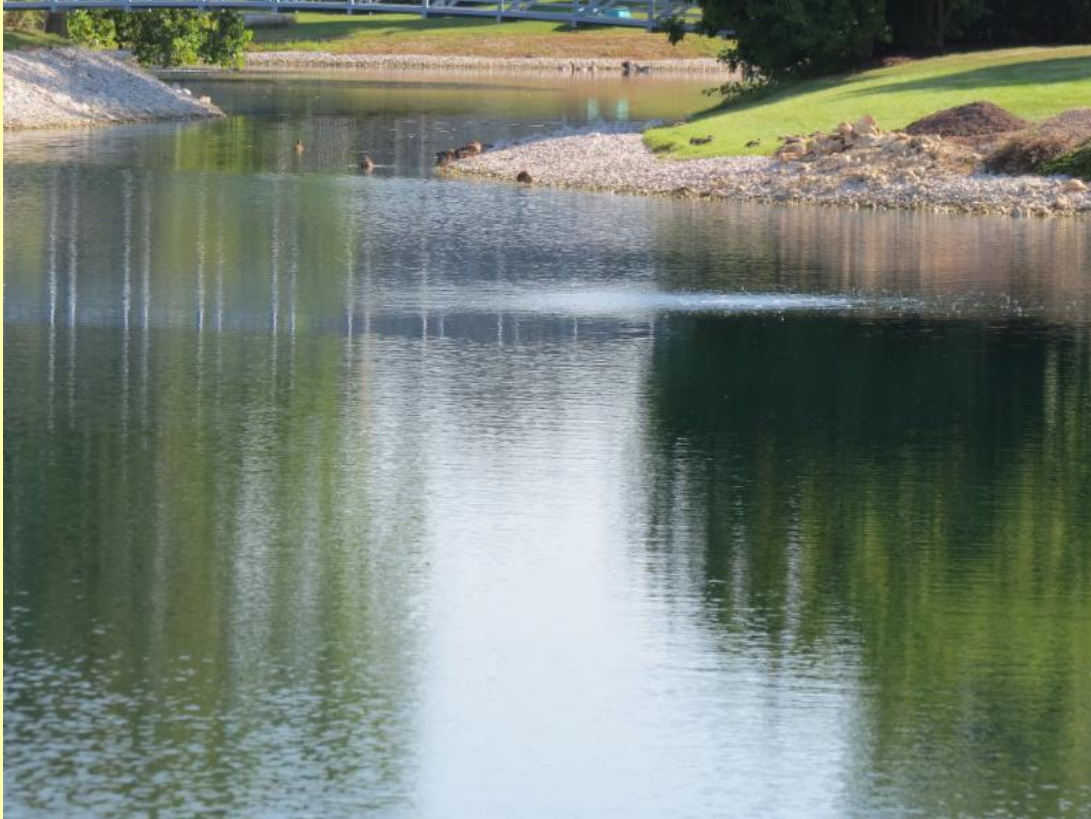
The shore of the pond was replaced with #2 rock.
