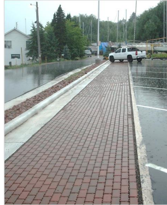
Permeable pavers/blocks-Bayfield, WI
