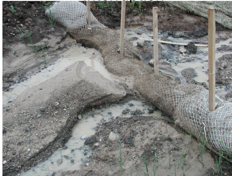
Manufactured Perimeter Control & Slope Interruption
