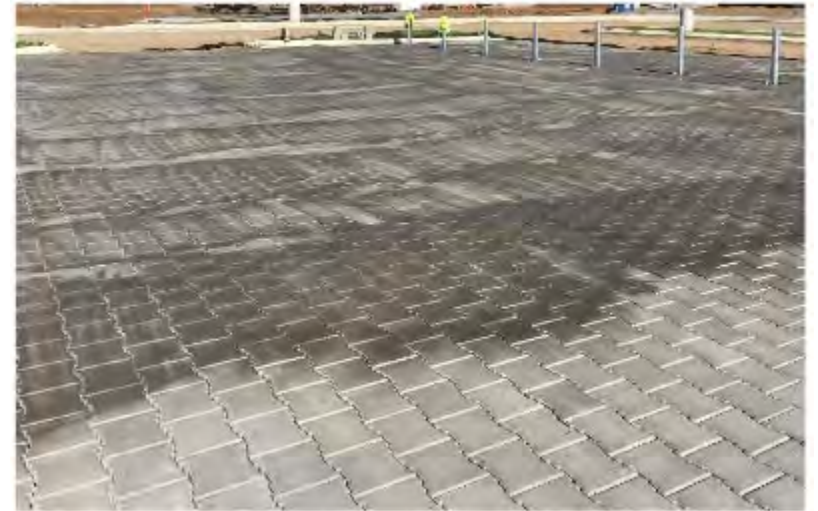
Close up immediately following sealant
