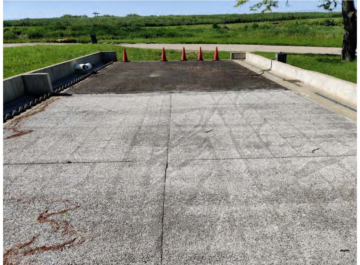
Permeable Pavement Testing Facility -East Side of Madison
