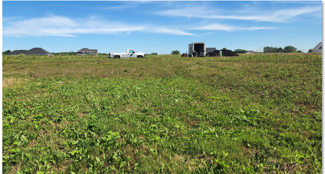
Basin that has been mowed too often and too short
