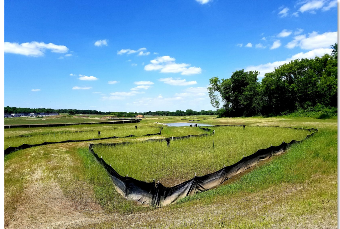
Infiltration basins the first spring after native seeding
