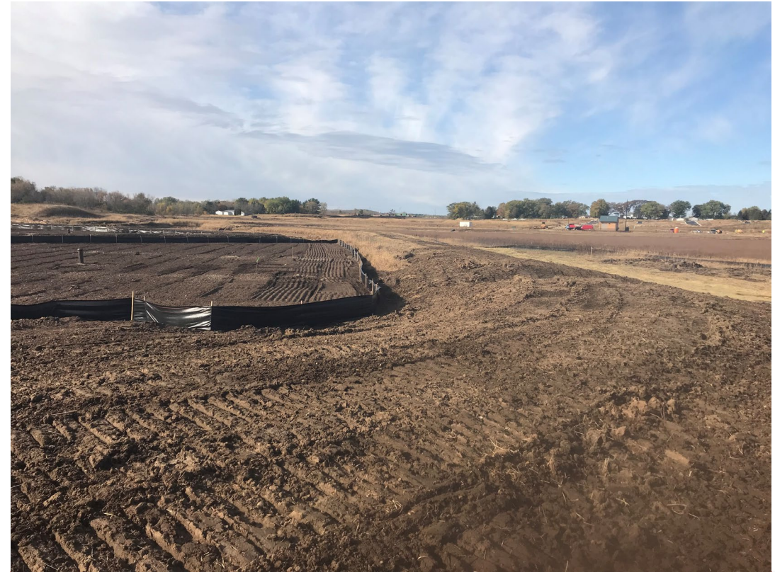
Final grading and soil prep inspection
