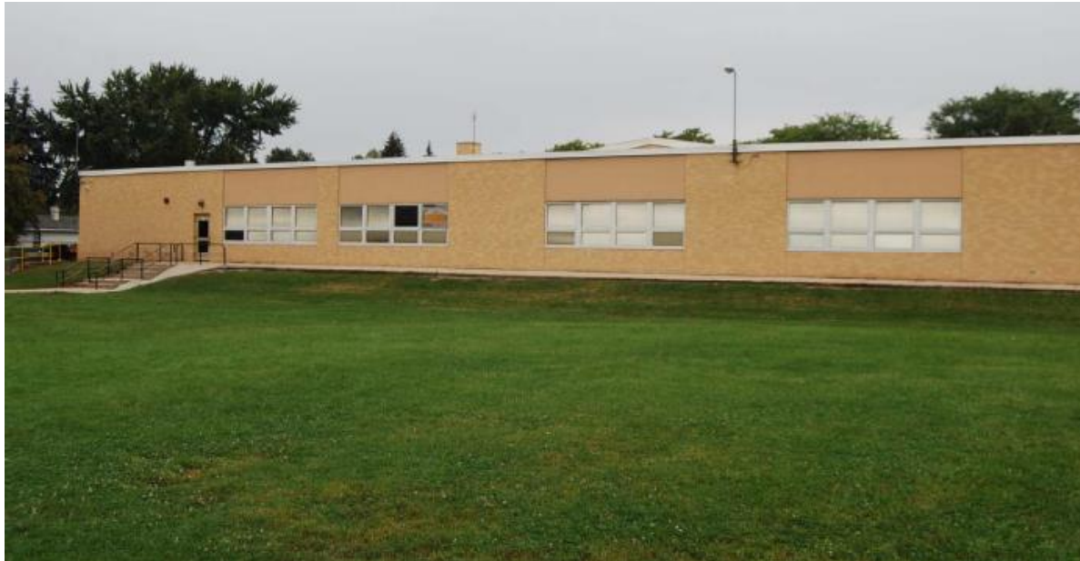
Areas of manicured lawn/paved areas
