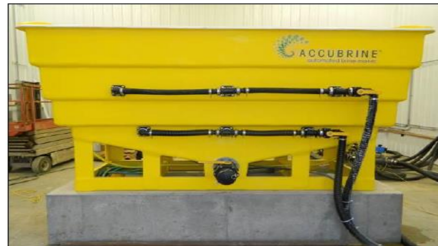
Accubrine salt tank on 2 ft concrete platform
