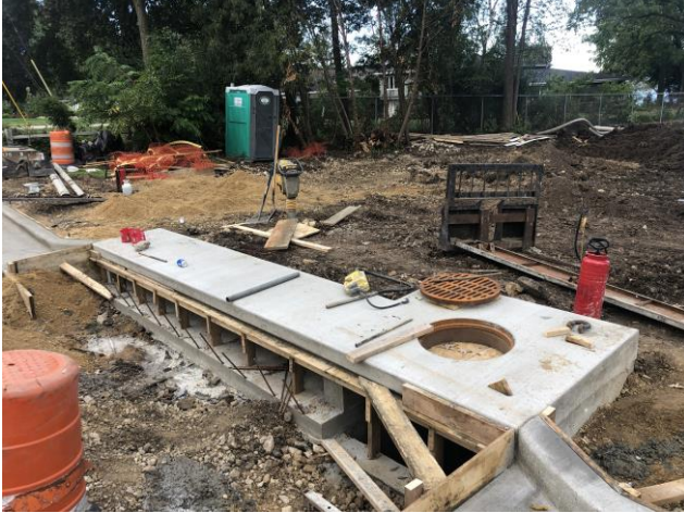
Open-throat high-capacity inlet
