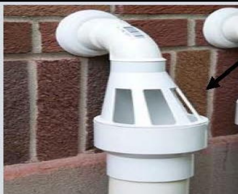
Freeze Protection Air-Gap
