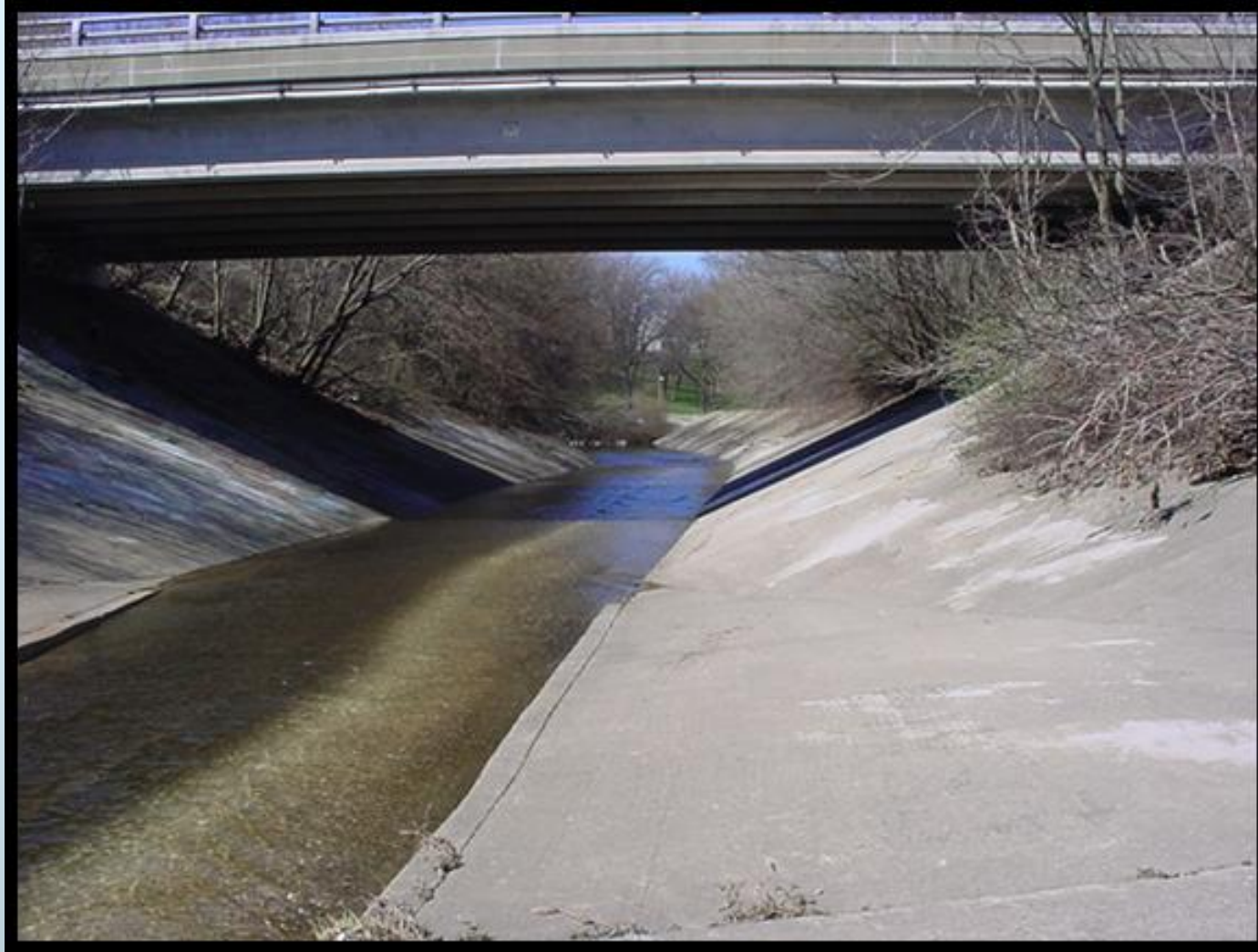
Upstream face of Cleveland #39
