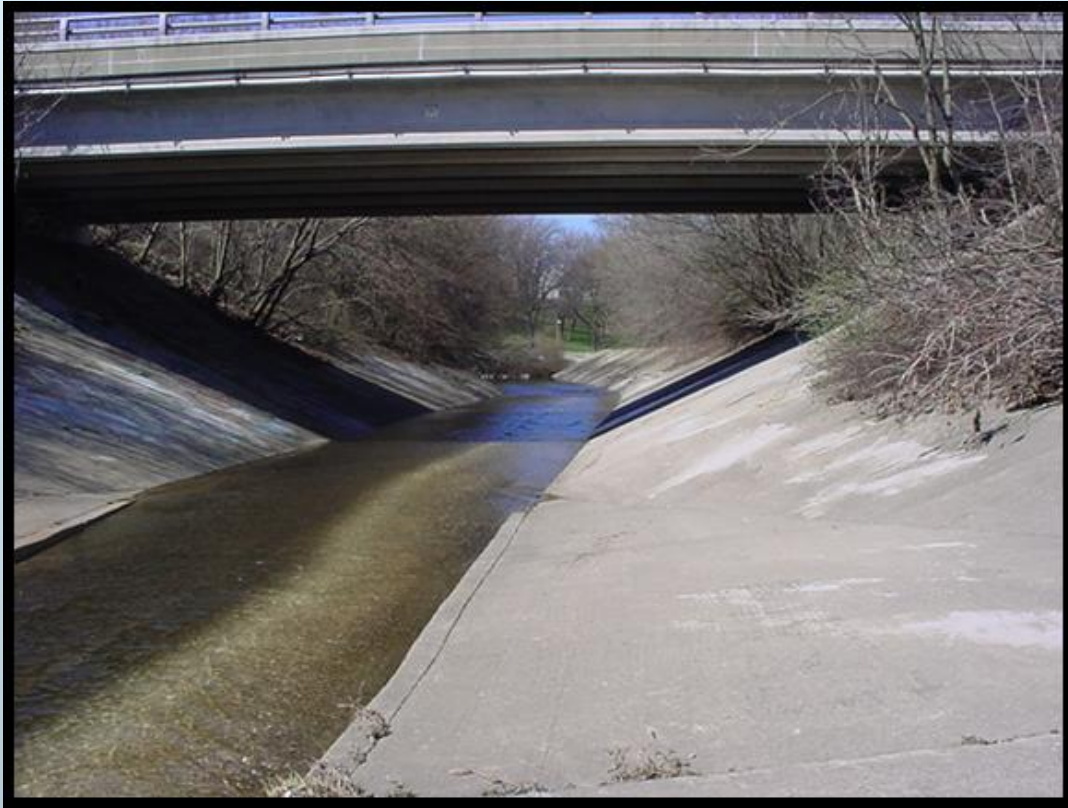
Upstream face of Cleveland #39
