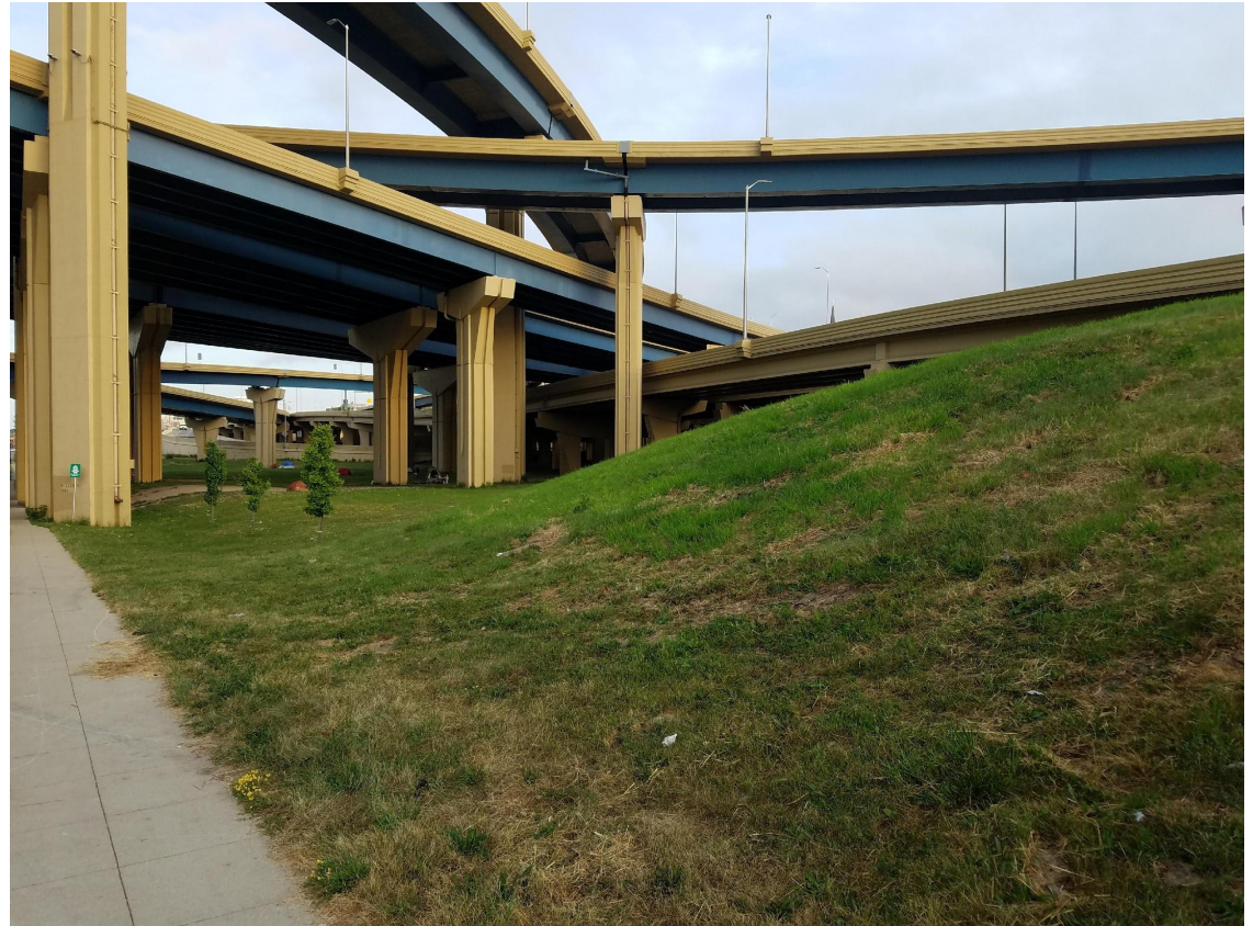
Preconstruction Marquette Interchange site along W St. Paul Avenue
