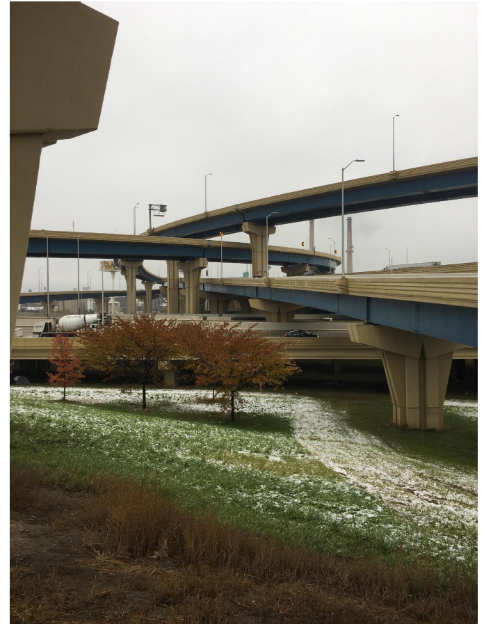
Preconstruction west site, facing south
