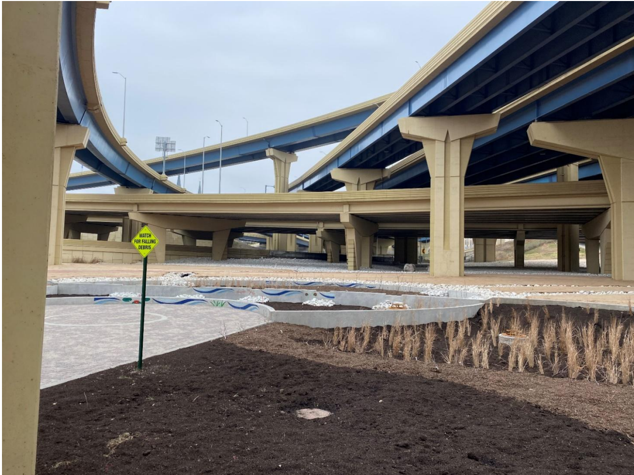
Completed bioretention basin on west site
