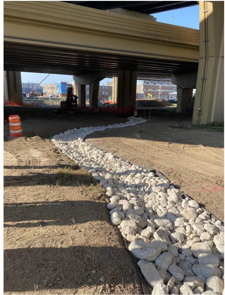
Rock-lined channel flowing to west bioretention basin
