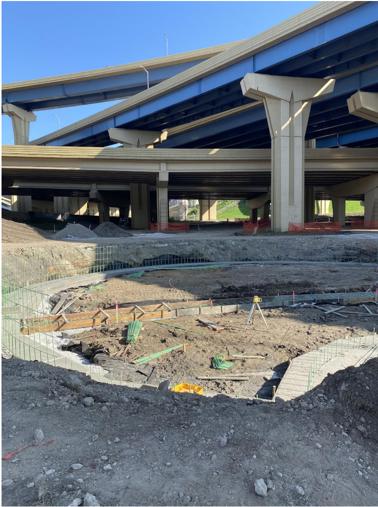
West bioretention basin under construction
