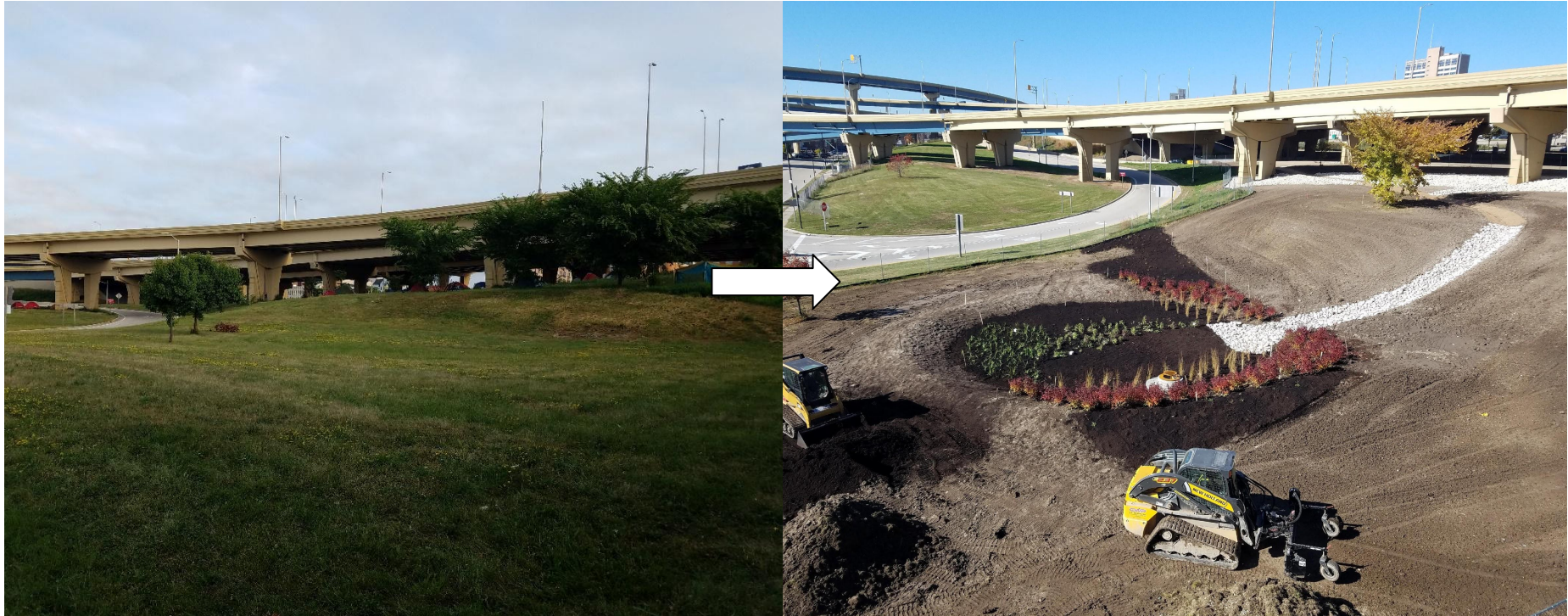
Preconstruction east site
