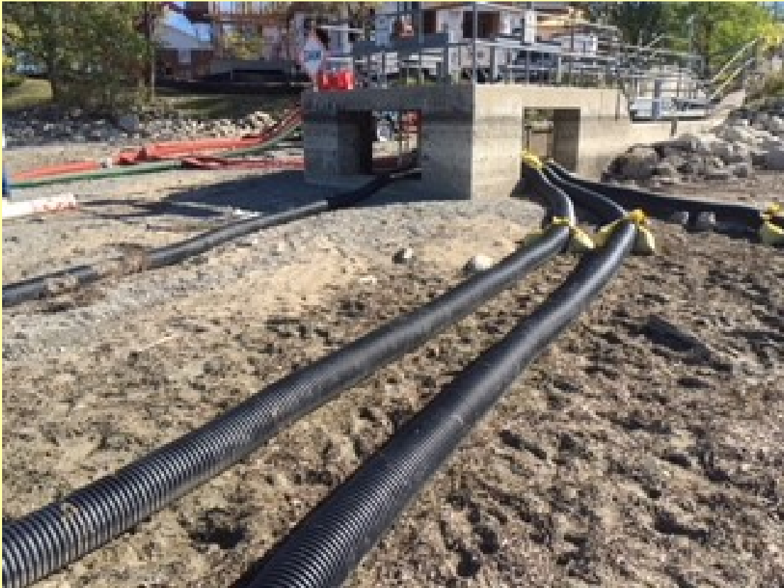
Water was pumped from the lake out through the dam. Photo: Brad Steckart
