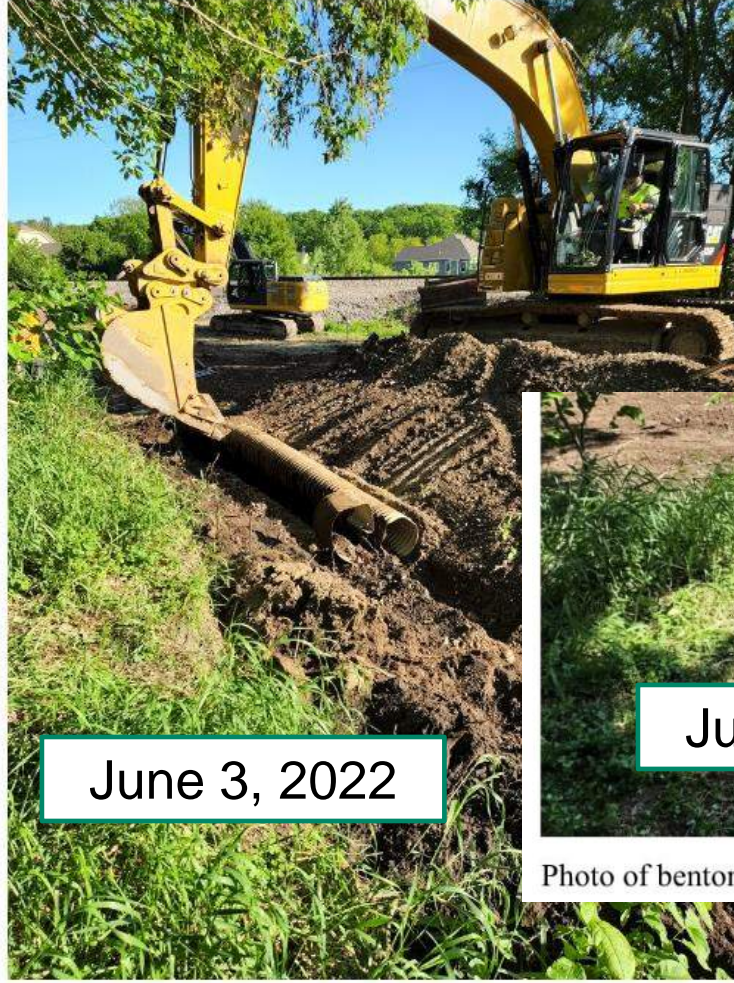
Photo of the removal of the existing 15" CMP just west of Springdale Road.
