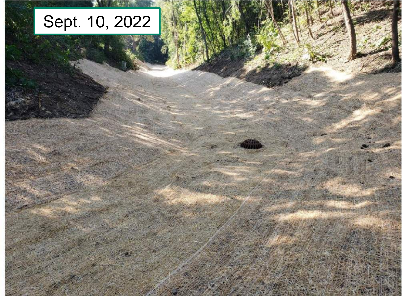
Final seeding and matting between MH1 and MH2 (closest).
