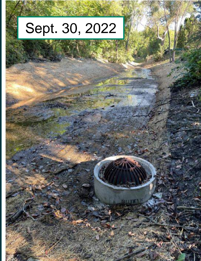
MH 1 looking north. Four bolts still missing from casting.
