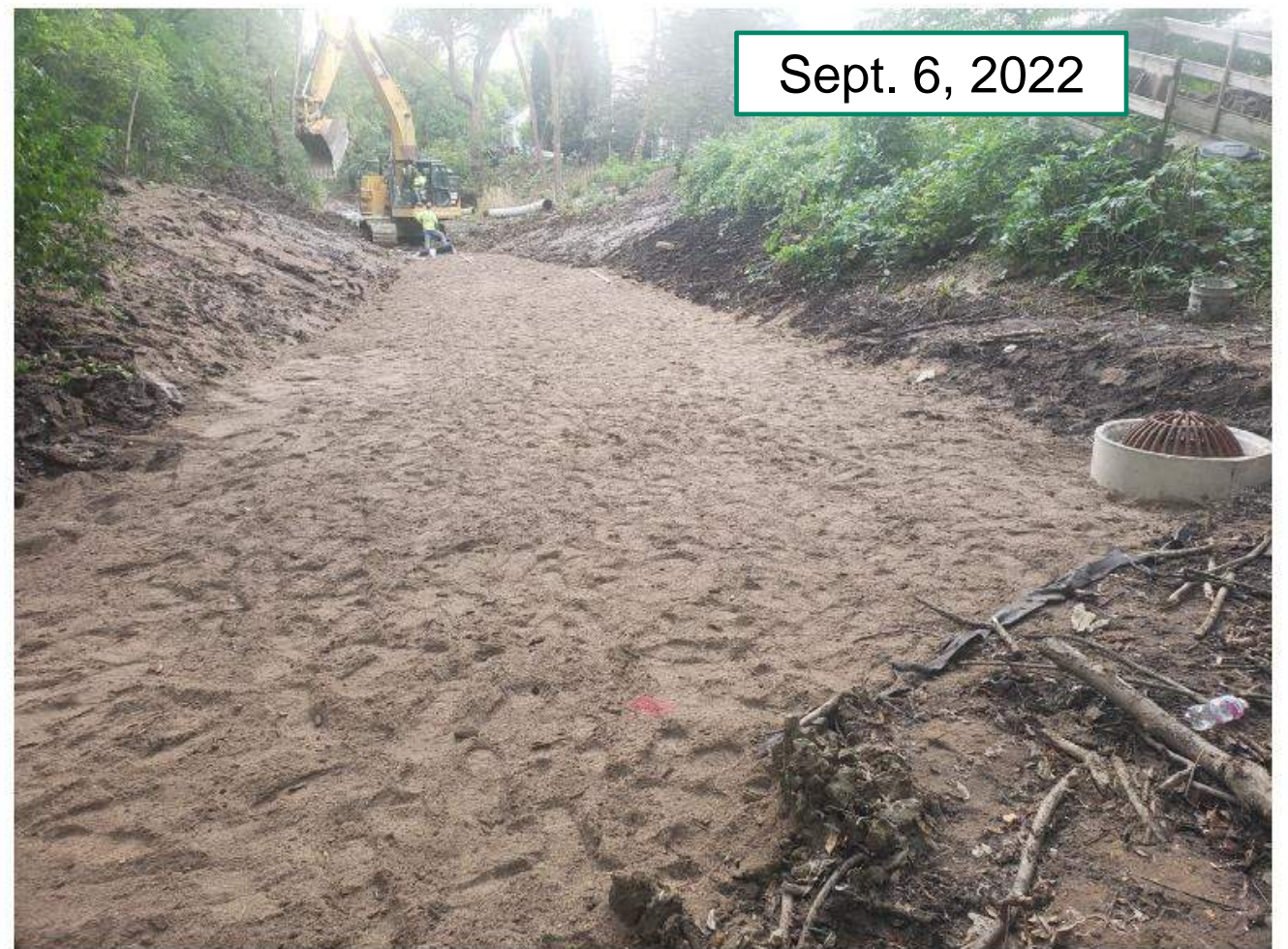
Engineered soil graded near MH1
