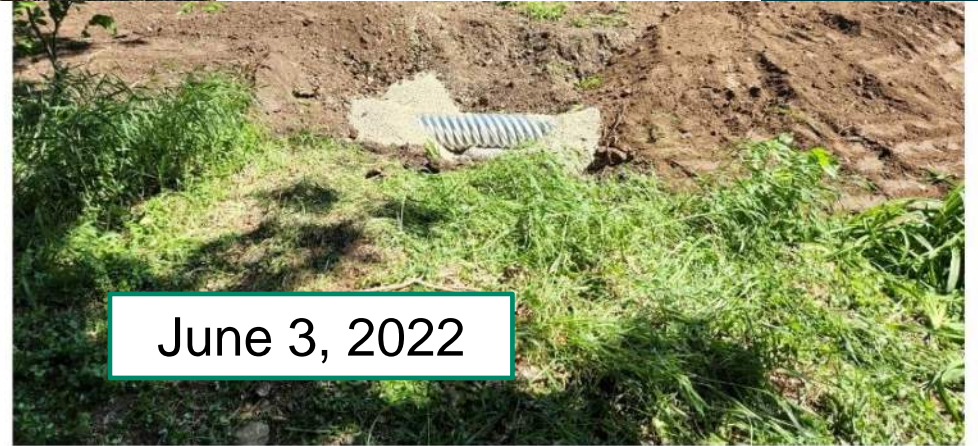
Photo of bentonite collar area, BP needs more material for sides and top of CMP.
