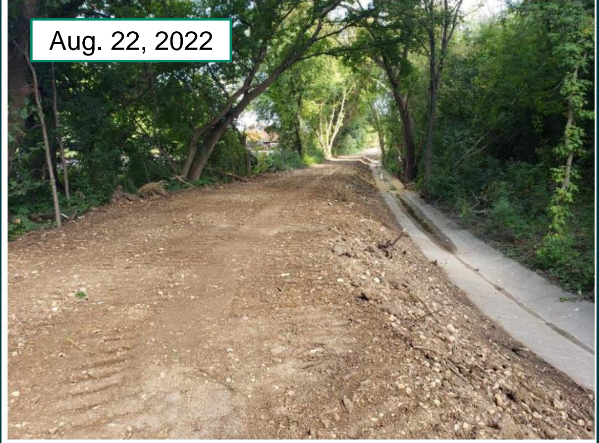
Leveled out soil after blasting between STA 5+50 to 7+50 (MH3 to MH4).
