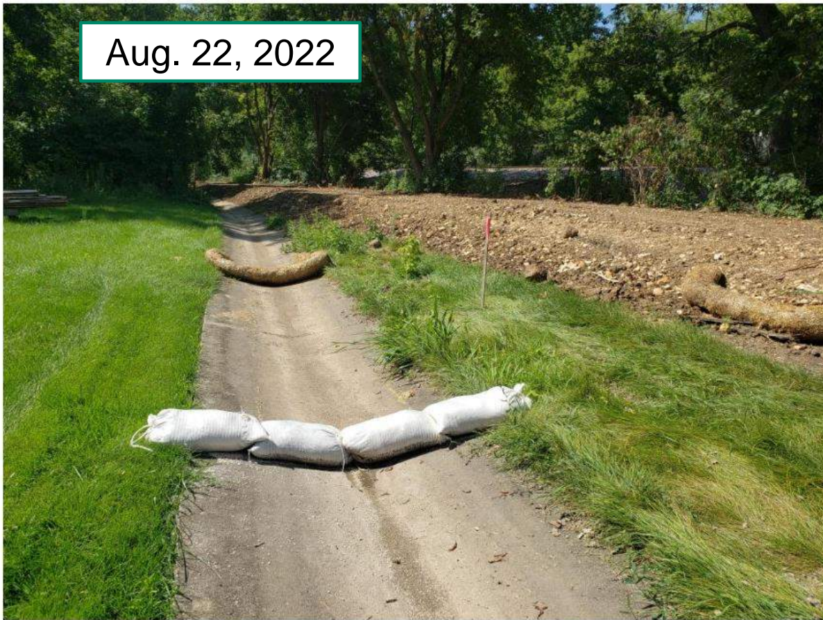
Installed erosion log downstream across concrete flume at ~STA 8+00
