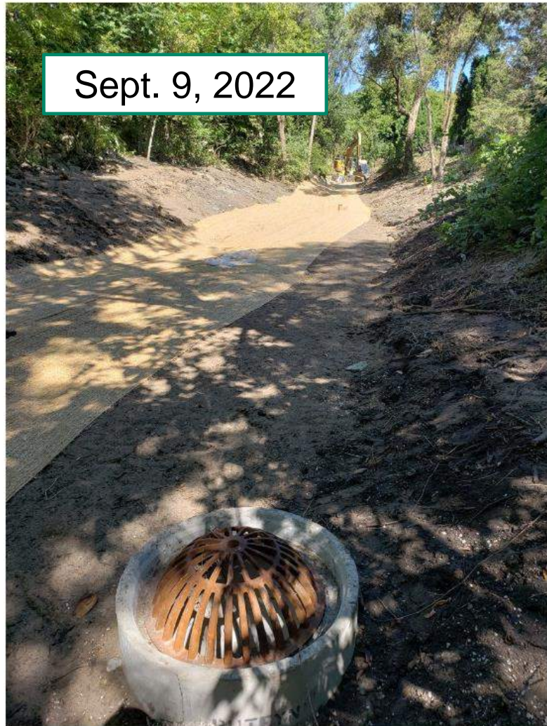
Progress of seeding and matting between MH1 and MH2
