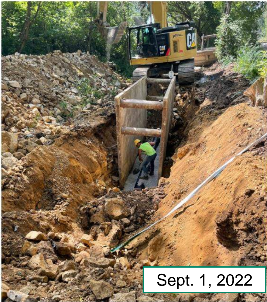
Installing storm sewer
