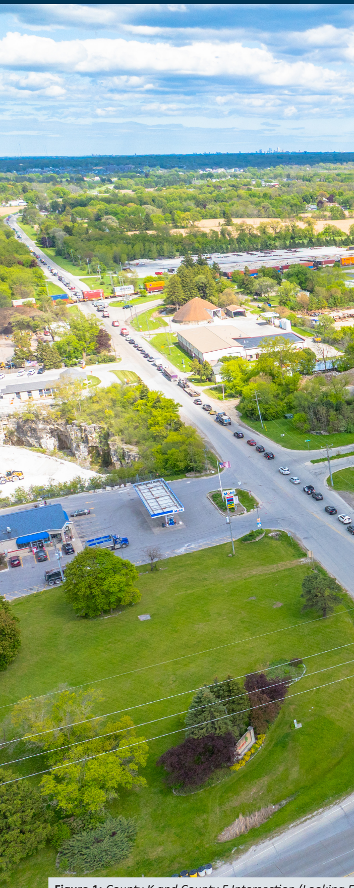
Figure 1: County K and County F Intersection (Looking East) – CN Railroad Crossing
