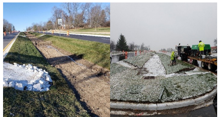
Figure 6: Waukesha County – County M Bioswale Construction
