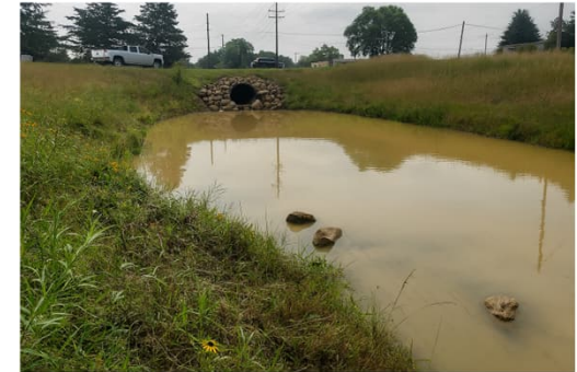
Industrial Park Dry to Wet Pond
