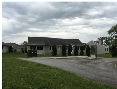
Submersible stormwater pump station
