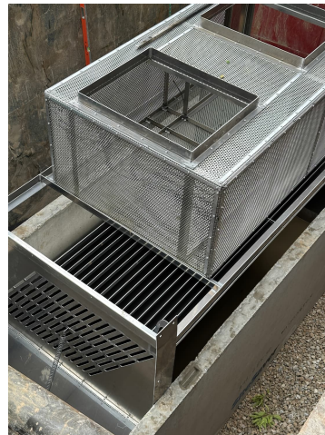
During construction (StormTrap Site Saver with Lamella Plates)
