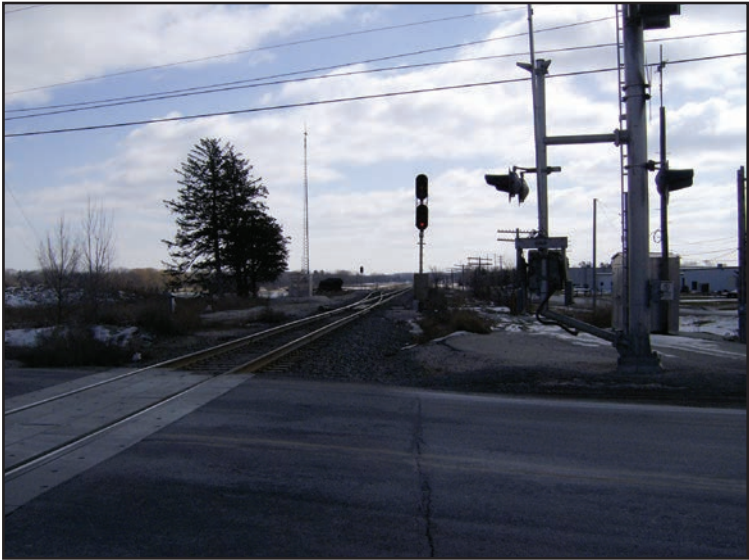
CN Siding Track Looking South at CTH K (Lisbon Road)
