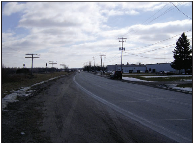
Duplainville Road Looking South Just South of CTH K (Lisbon Road)
