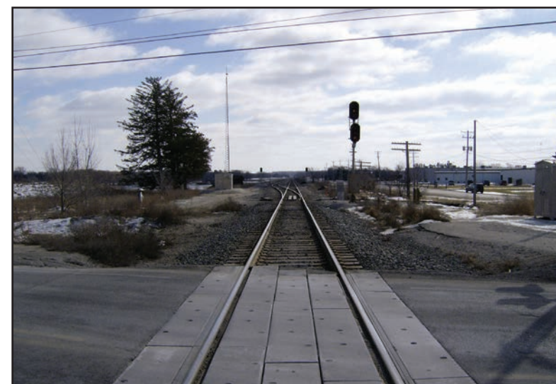
CN Mainline Track Looking South at CTH K (Lisbon Road)
