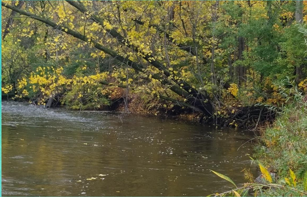
Failing bank and scour pool
