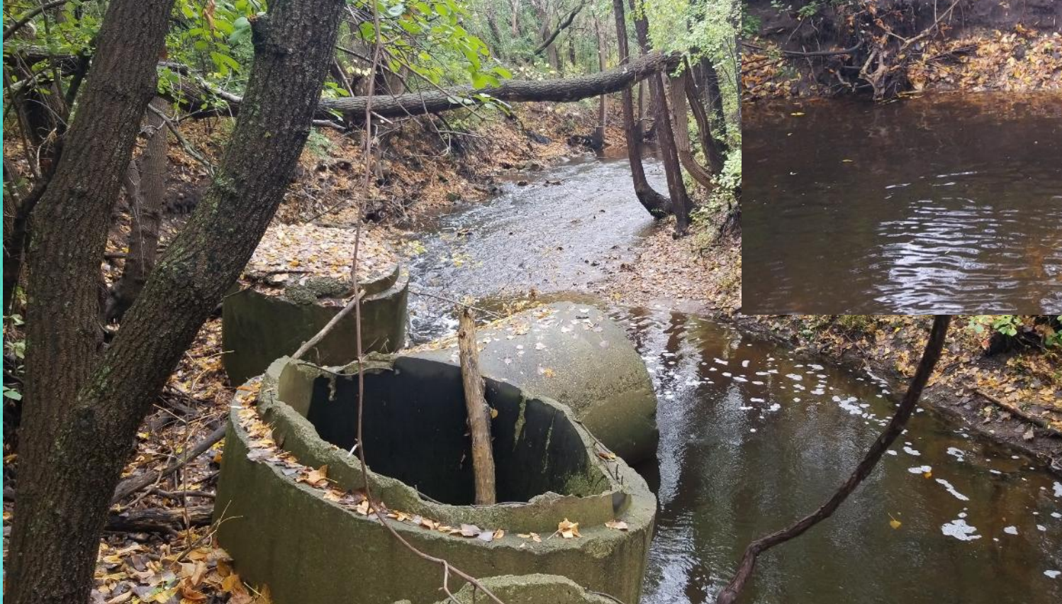
Failed revetment
