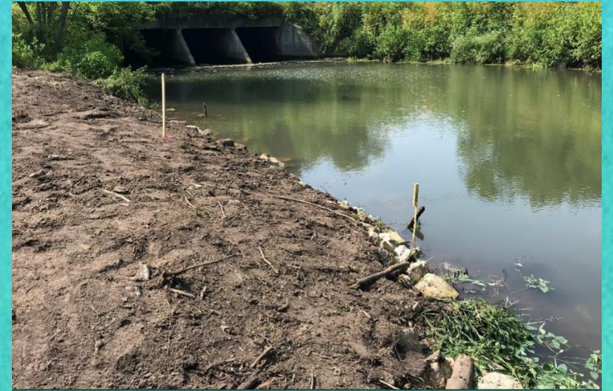
Vegetated Boulder Toe w/ Bank Grading
