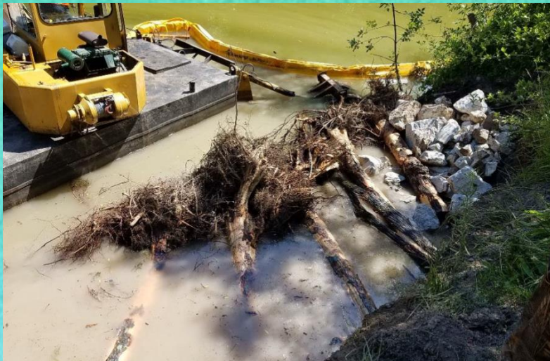
Rootwad w/ Stone Revetment
