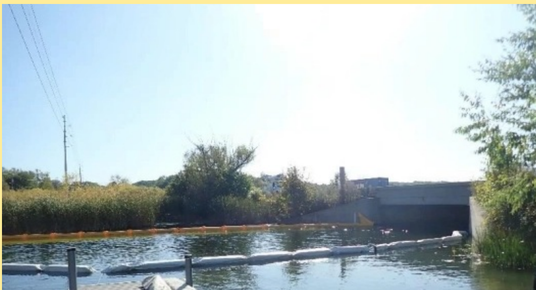
Silt curtains to contain fragments of plant material (Photo credit DNR)
