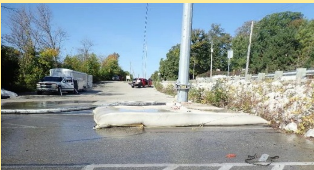
Geo-textile bags that collect plant material and sediment (Photo credit DNR)
